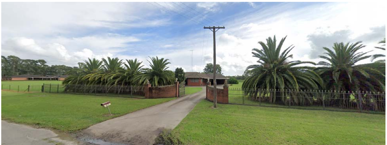
Figure 4 39-45 Old Castlereagh Road, as viewed from Castlereagh Road (Source: Google Street view)
